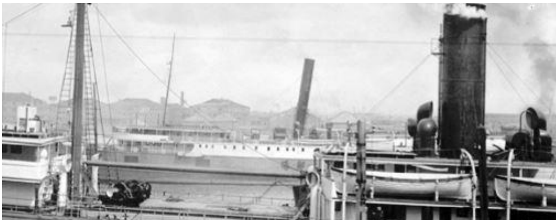
POYANG, showing development of bridge structure (CNC/Wikiswire).
