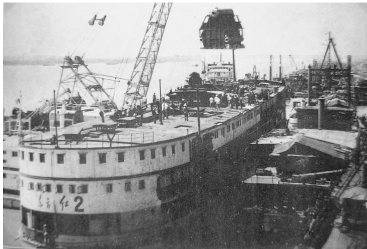
DONG FANG HONG 2 under major refit, evidently receiving a new main boiler. Stern plating/porthole arrangements match YOHYANG MARU identified by LR as CHIANG HAN ( The Yangtse River ).
