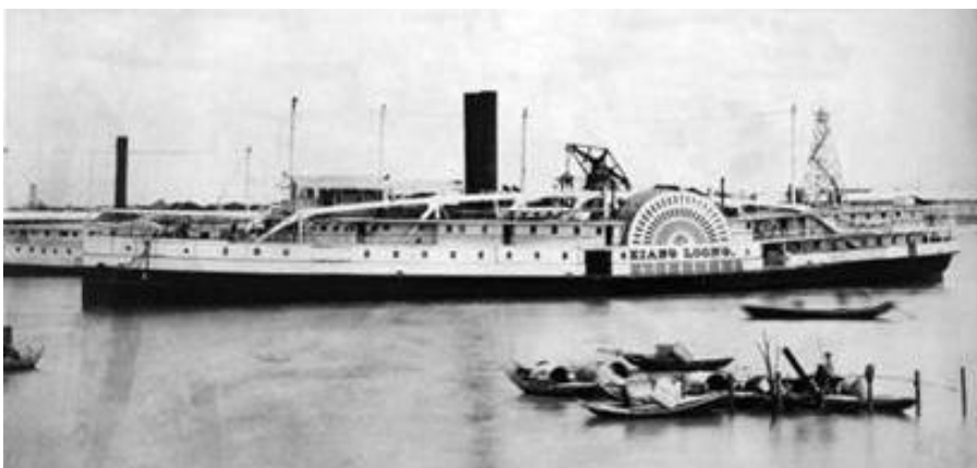
SZECHUEN's origin KIANG LOONG showing Neptune-made "walking beam" of engine (Internet).
