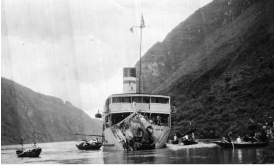
LOONG MOW being refloated in the Gorges with bow damage after colliding with a cliff on 14/7/20 (Capt. John Dewar).
