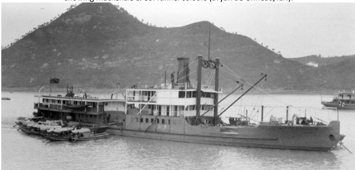
WANHSIEN with a cut down superstructure at Ichang (Warren Swire colln).
