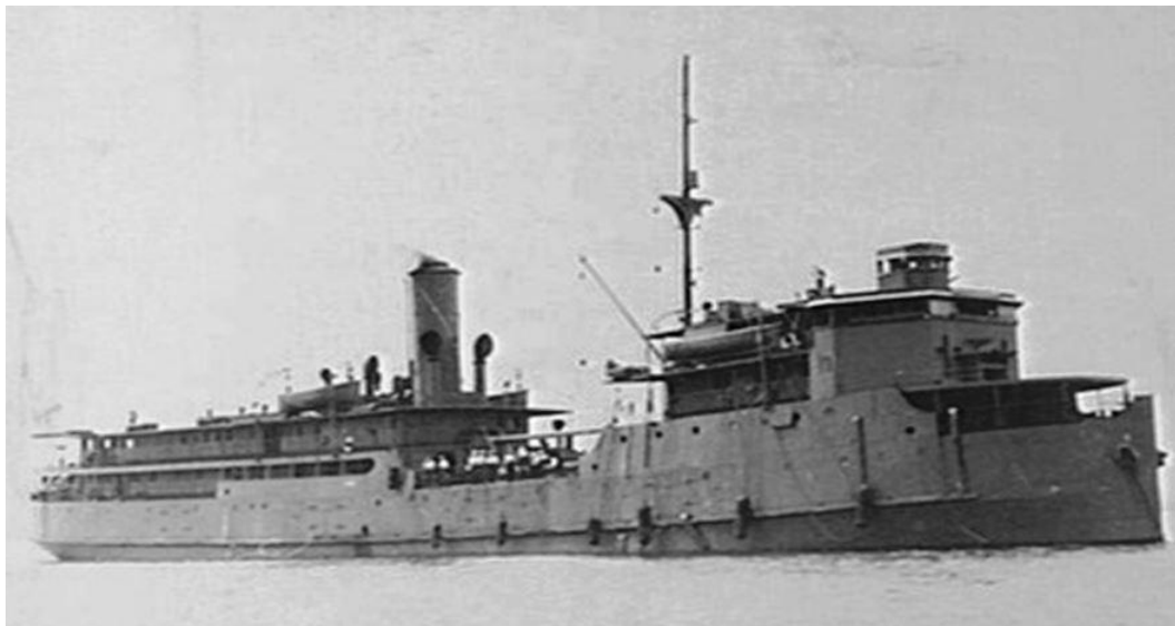
HMAS PING WO in early 1940s. Front bridge corners removed by R.N. to improve firing arc for 12-pdr gun, later dismantled (as here) (M Neg No.301177).
