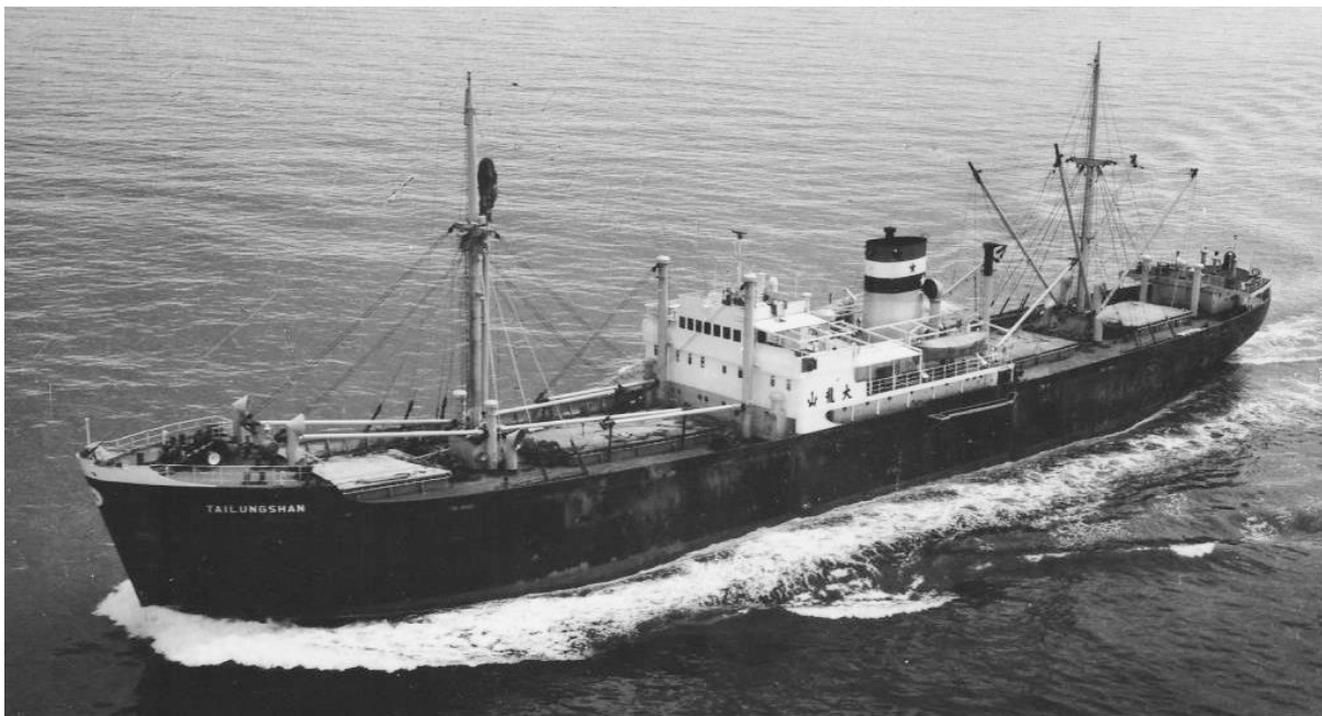
Refitted, including two new kingposts aft of superstructure (P. Foxley/SK*).
