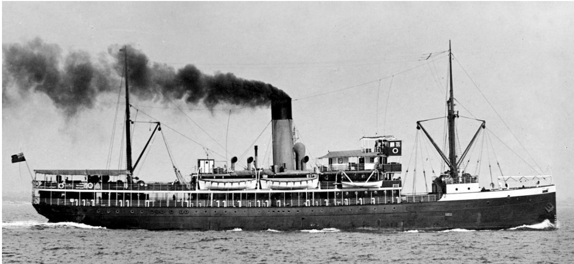
HAI LOONG before acquisition as Adelaide S.S. Co. MORIALTA. As built with low fo'c'sle and flying bridge plus radio aerials (A.C. Green/State Library of Victoria).
