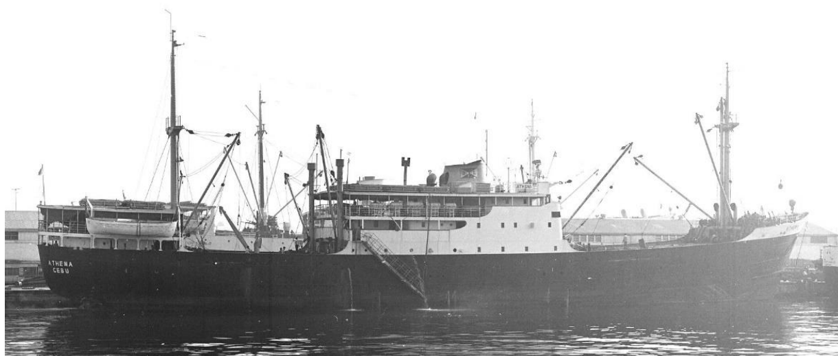
ATHENA, Manila North Harbor, 3 June 1970, new awnings, rafts replacing boats (W. Schell).
