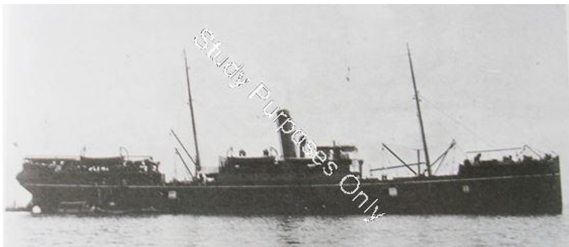
HAICHING at Singapore on charter after 1929 refit. Mainmast moved forward and kingposts fitted between Nos. 1 and 2 hatches (KPM Archive/Alg. Rijksarchief).
