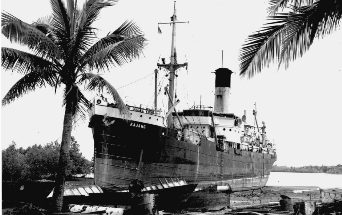
KAJANG (1916) beached for demolition by Hong Huat, mid-1960 (R. Gabriel/H. Dick*).
