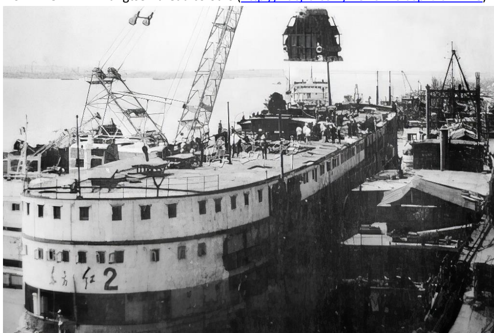
DONG FANG HONG 2 receiving post-1966 boiler replacement at Wuhan ( The Yangtse River ).
