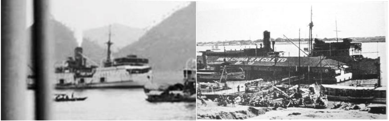
PING WO at Ichang in 1926, and in the late-1930s on the outside berth at Hankow. Superstructure now closed in forward and extended aft, but still good facilities for cargo-carrying (L: John Swire & Sons, R: China Proper Vol III ).
