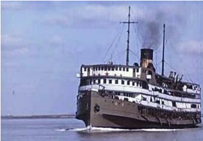
Photo, thought to be of rebuilt CHIANG SHUN, with revised bridge and mainmast newly fitted ( http://ayuczds.blog.163.com/blog/static/22154207320135173213612/ ).
