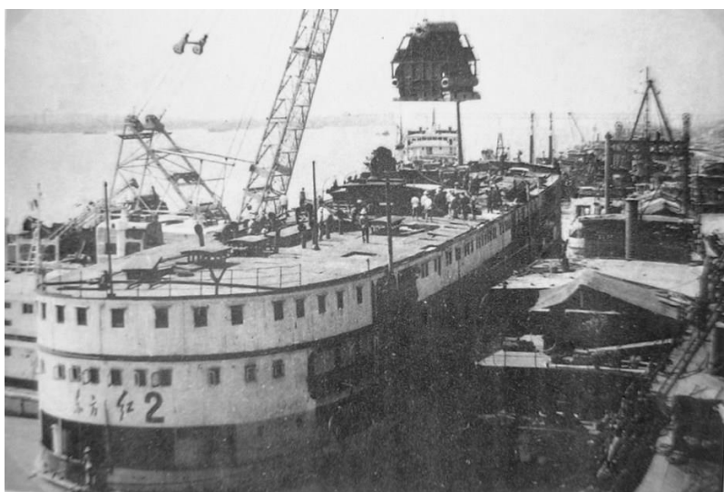
DONG FANG HONG 2 under major refit, evidently receiving a new main boiler. Stern plating/porthole arrangements match YOHYANG MARU identified by LR as CHIANG HAN ( The Yangtse River ).
