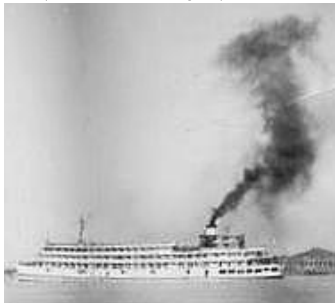
DONG FANG HONG 9. Hatch removed, top deck built up, funnel raised one deck (7788.com).
