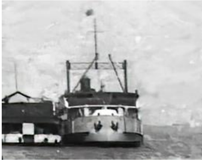
Bow view of PAOWO at Hankow showing cargo gear atop superstructure (kongfz.com)
