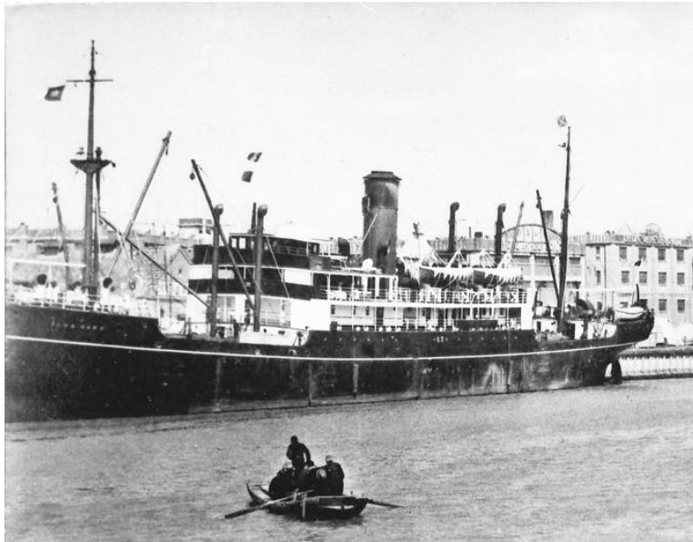
TINGSANG (TING SANG on hull) Tianjin 1930s, new anti-piracy barriers visible at front and rear ends of superstructure (from a postcard in Yoshihide Kobayashi coll.).
