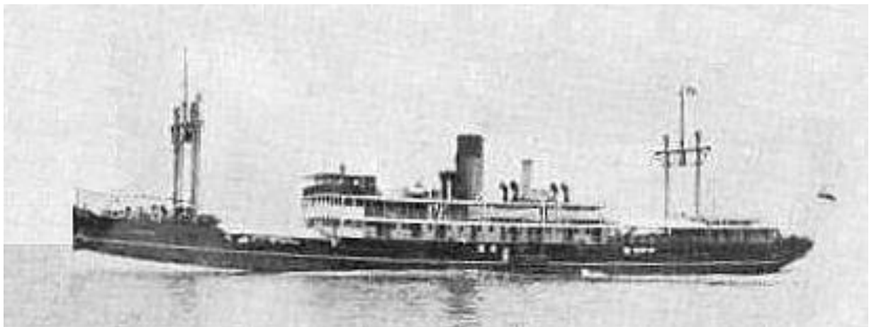
LIENSHING heavily laden, with deck awnings, canvas vent, and re-angled cowl ventilators (SK coll).
