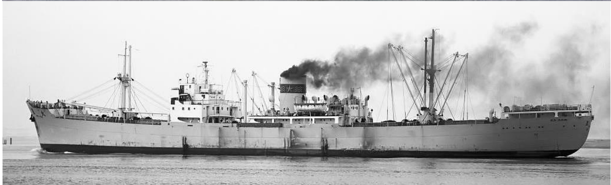
XING HUO ex HOPING 54. Further update to wheelhouse, superstructure front enclosed for extra accommodation (B&W photos at Rotterdam 21 June 1970 Malcolm Cranfield).
