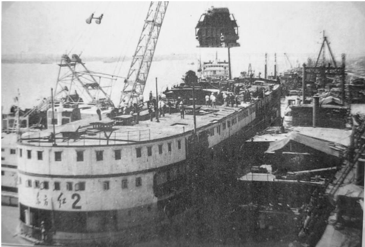
DONG FANG HONG 2 ex-YOH YANG MARU under major refit in 1966, evidently receiving a new main boiler ( The Yangtse River ).
