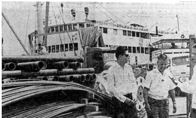
Rebuilt superstructure of (readable) RAJAH SULIMAN ( Manila Times 28/6/67 SK).
