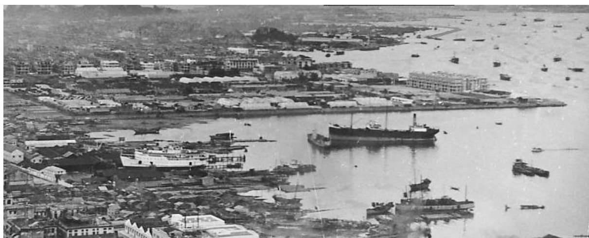
TAI LOY on the slipway in 1950 (Henri Cartier Bresson).
