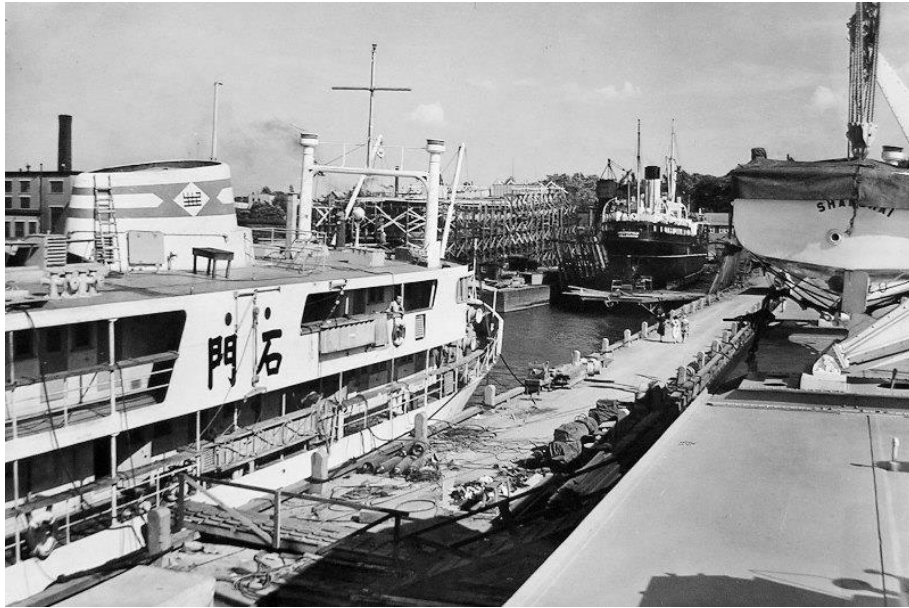
900 grt SHIH MEN of Ming Sung nearing completion at Lauzon on the St. Lawrence River (SK*).
