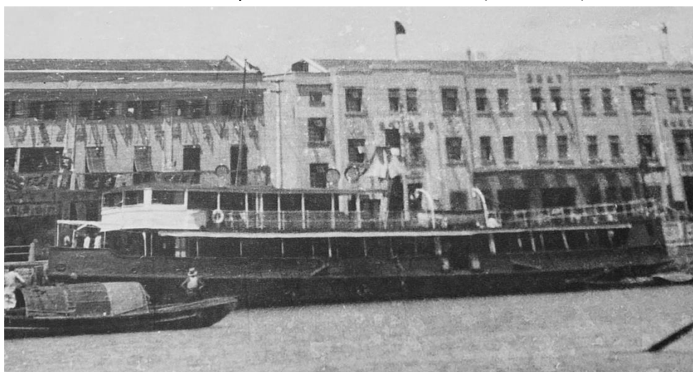
Assumed TSZPEH alongside at Ningpo 1934 with bridge structure extended aft and stern plated in around the upper deck (Wang Zhi-Xiang/Ningbo Museum).
