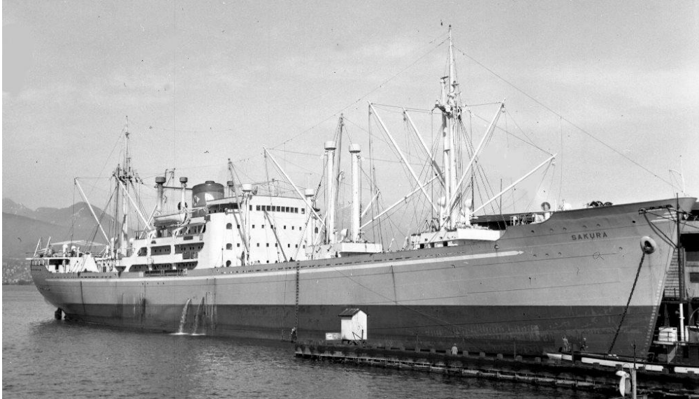
SAKURA at Vancouver c.1951, rear kingposts now joined (Ken Thompson/W. Schell).
