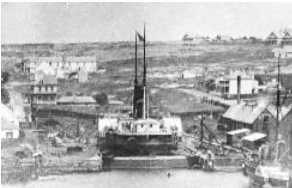
NEVADA under repair in Mort's Dock, Sydney 10/71 (ANMS0031[052]).
