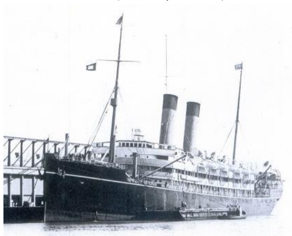
KOREA as T.K.K.'s KOREA MARU showing open plating on port side of main deck (Noma & Yamada).
