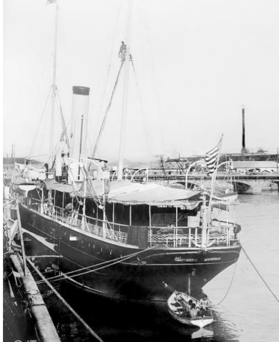
Refitted TAN-AUCO ex BANJERMASIN below Bridge of Spain, Pasig River, Manila, c.1900 (Univ. of Michigan).
