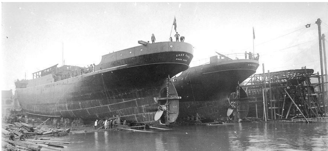
CHAK SANG being prepared for launch at Kowloon. PROSPER adjacent (HK&WD/HKMM ID2008.0197.019b).
