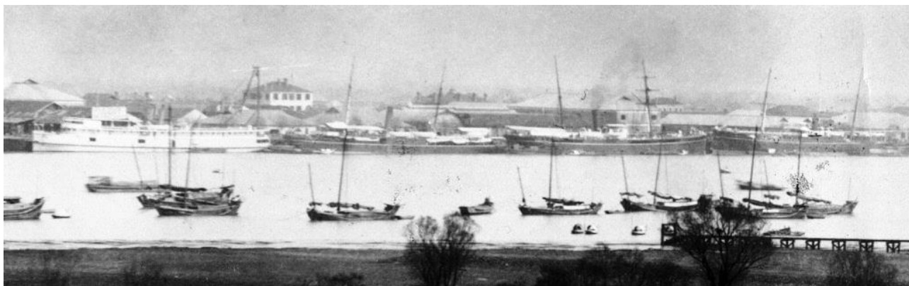
Four Jardine steamers at the Hongkew wharves in Shanghai on the early morning of Tuesday 31 March 1891. From left, TAI WO discharging from Lower Yangtse ports, KOW SHING loading for a late afternoon sailing for Ningpo, FOOKSANG about to sail for Swatow and CHOY SANG loading for a 2 April sailing for Chefoo and Newchwang (Kung Tai/UoB dh-s130).
