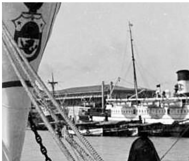
Late photo suggests installation of new railing protection and prominent awning above superstructure (Robert Pendleton/UWM).
