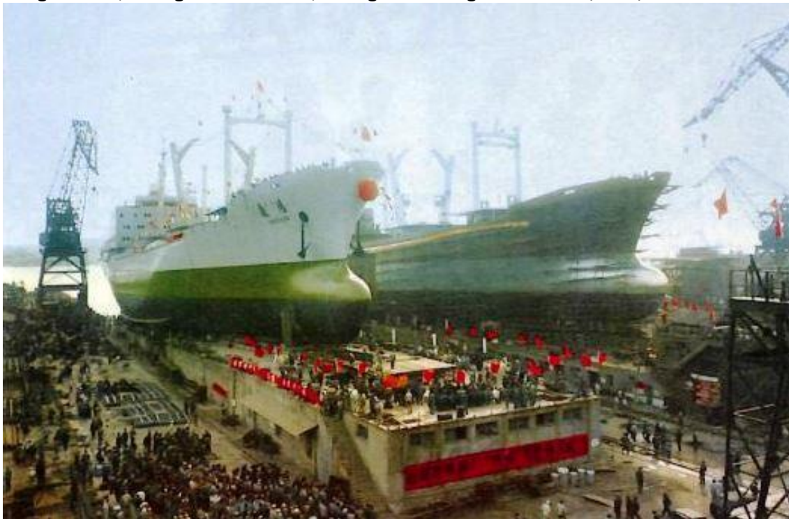
Launch of QING YANG. YI YANG to port ( China Reconstructs 7/72).
