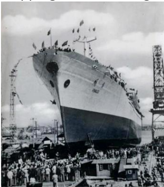
FENG LEI at at launch and completion, only 'FENG' ship without a bulbous bow (Shanghai S.Y.).
