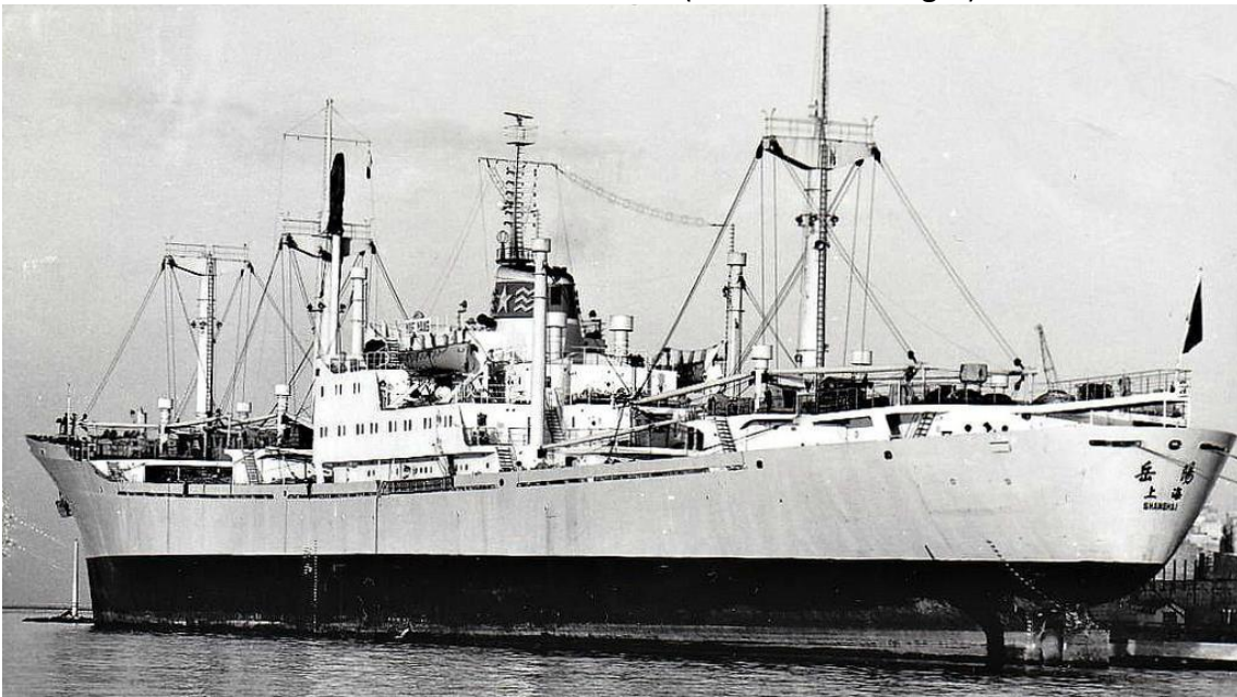
Only GAO YANG/XIANG YANG and YUE YANG (above) had a knuckle along the fo'c'stle (coll. SK).
