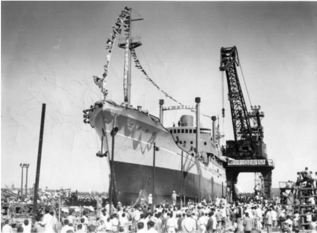
ZHE HAI 1 being launched by Zhonghua Shipyard (Shanghai) in 1960. This only photo, yellowed with age, was bought on a Chinese internet auction site nearly 60 years later (SK*).
