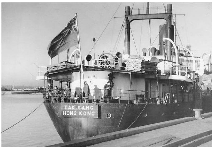
TAK SANG with removable nameboard, evidently re-shortened funnel, presence of military personnel, and absence of hull band in an unsourced photograph dated 12 March 1939.
