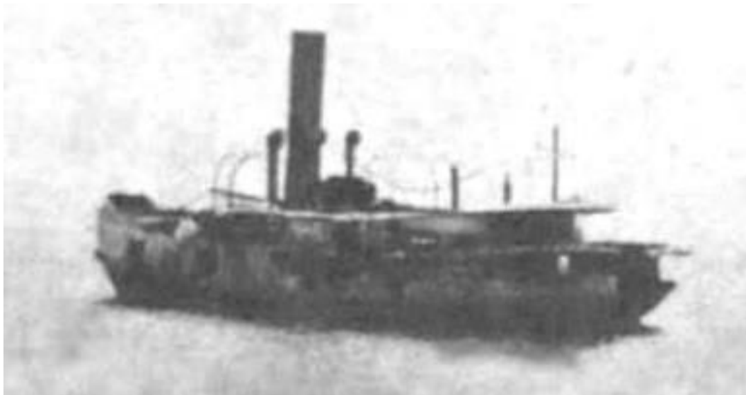
TA CHIE after gutted by fire on 11 March 1931 ( http://60.250.180.26/ss/6285-2.html ).
